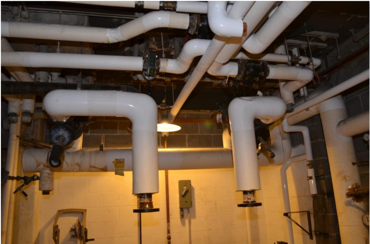
Of course, in buildings as old as Jones Hall, asbestos was used for a lot more than just coating floors and tiling, it was also used as insulation for piping (shown above), meaning that it can potentially be found anywhere and everywhere inside the walls. Making sure asbestos doesn't escape and create a serious environmental hazard requires a lot of internal demolition. AT checks every wall for signs of asbestos and
